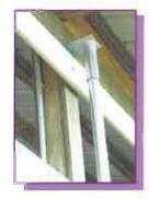
Standard 2" GatorShield structural 14 ga pipe used to make all vertical curtain retainer tracks.
