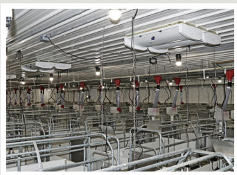
DL3232 Insulated Air Inlets Installed in Hog Barn
